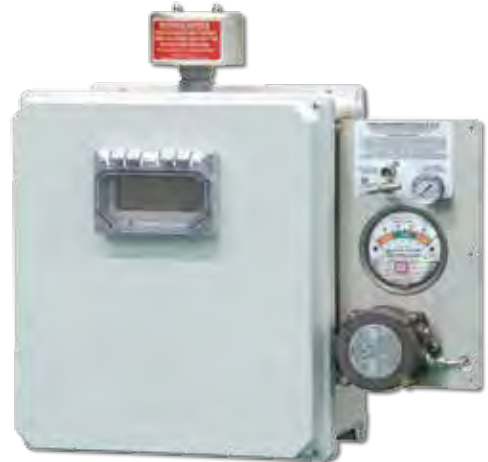
Weigh-scale display and controls in the hazardous area with Bebco EPS 3000 Type Y purge systems
